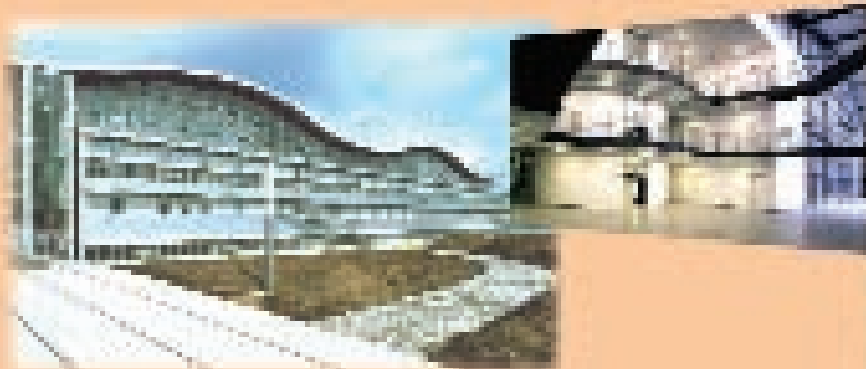
IPP Greifswald building (Wendelstein 7X)
