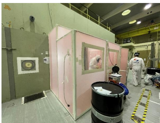
Ispra-Decontamination of hot cells in LCSR
