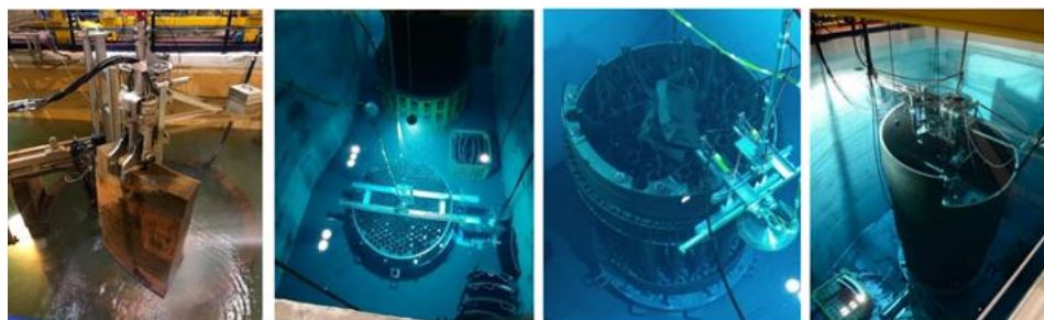
Figure 3: Cutting of Reactor Pressure Vessels at Bohunice
