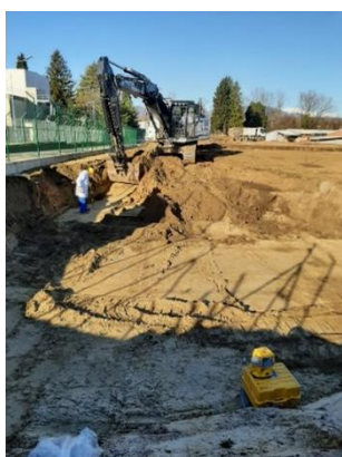
Ispra-Retrieval facility excavation work yard
